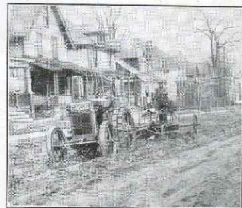
Case 10-18, rubber tired, grading an unpaved street
